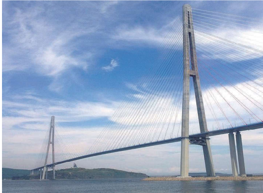
Figure (1.1) The world's longest cable-stayed bridge, Russky Bridge (1 104 meters), Russia.[4]
