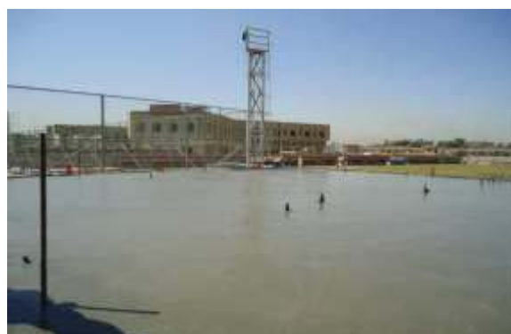
Plate (1-12): Foamed concrete for using roof in Sports AL-Ascan Club in Baghdad(Anadolu Construction Company)
