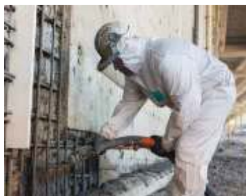
Plate (1-9) : maintenance of damaged concrete
