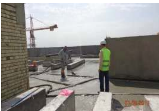
Plate (1-11): Foamed concrete for using isolation thermal in city of visitors in Karbala (Anadolu Construction Company)
