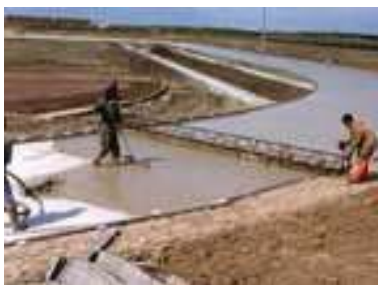
Plate (1-8): Fix settlement soil by Foamed concrete
