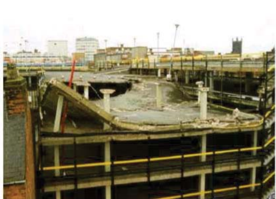
Plate(1-1): Piper's Row Car Park, Wolverhampton, UK
