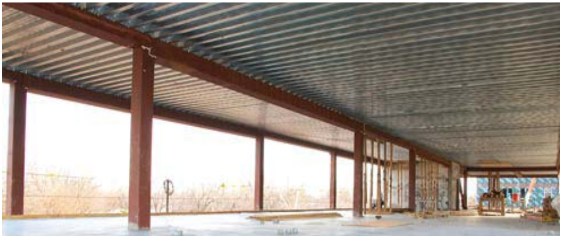
Figure(1-3) Building Consists of Composite Beams Provide Large Space (New Millennium Building Company) [33]
