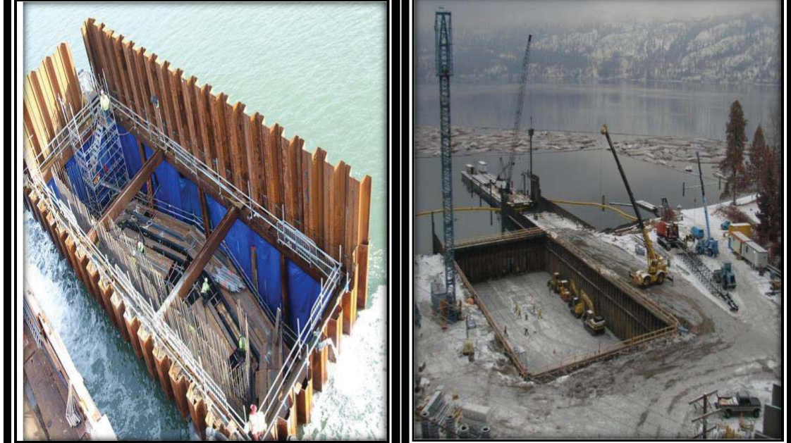
Figure (1.1): Sheet piling wall (design buildings, 2017).
