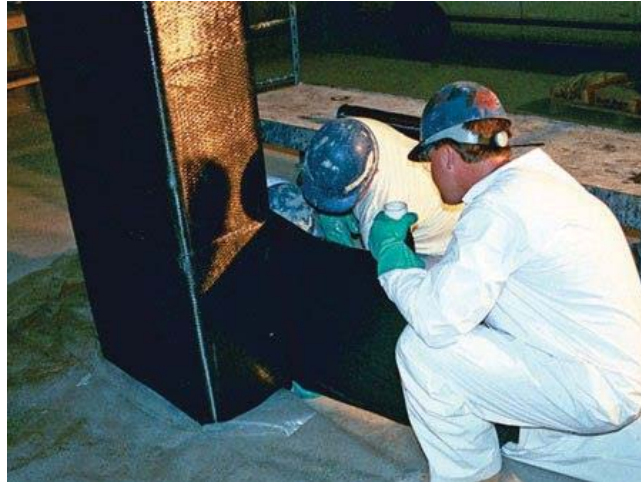
Figure (1-1): Jacketing of Columns by CFRP (Jijin et al, 2015).
