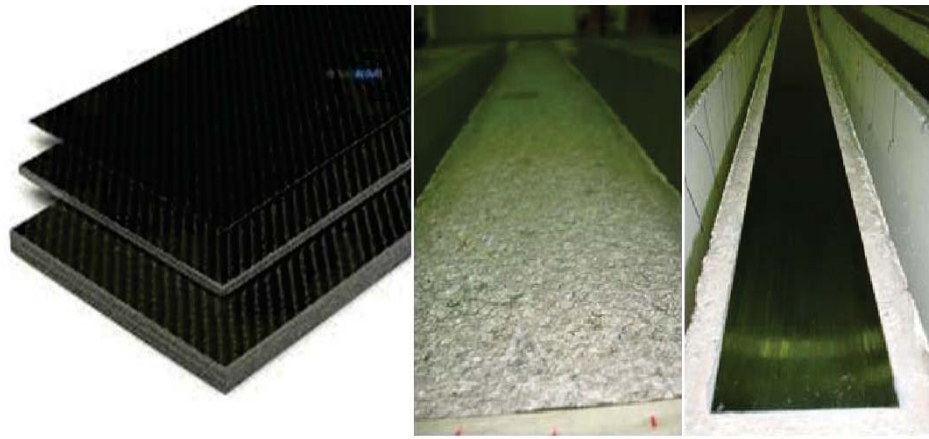
Figure(1.5)Surface preparation and CFRP fixing(13).
