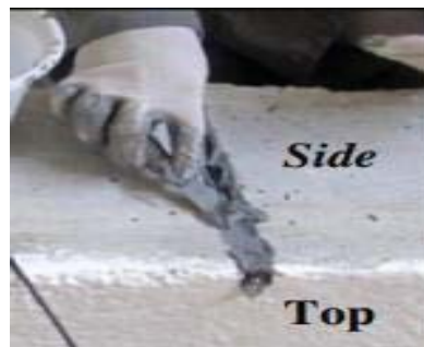
(c) Applying the epoxy adhesive for filling the grooves.
