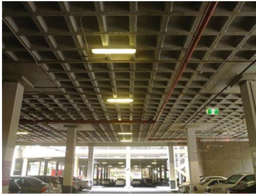
Figure 1-1: Waffle Slab molds (Al-Issawi, 2023)
