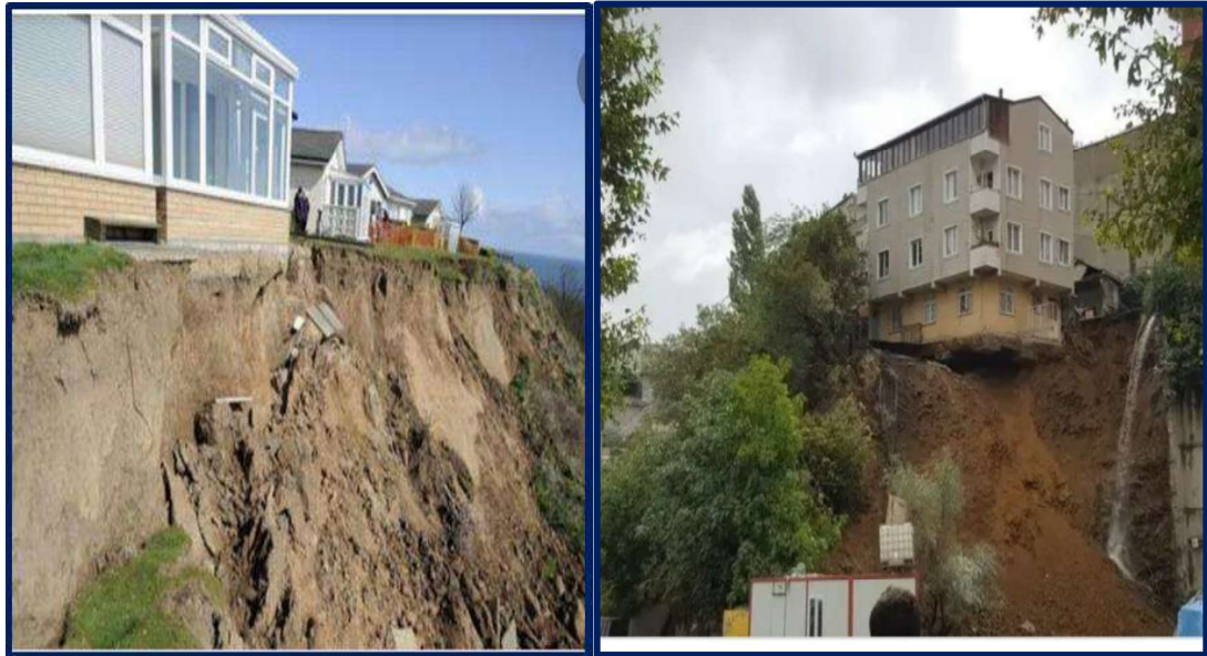
Plate (1.1) Failure of Buildings That are Built on Gypseous Soil (After Abid-Awn, 2010).
