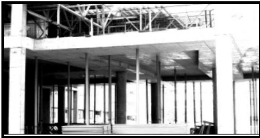
Plate (1-1): Toronto high-rise with wide beams building (Al-Mashhadani,2016).
