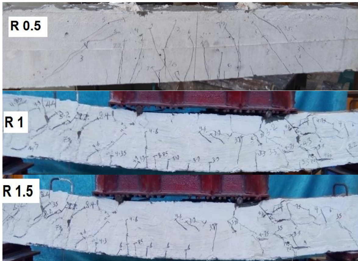
Figure 3. Mode of failure of beam at group 1 (G1)
