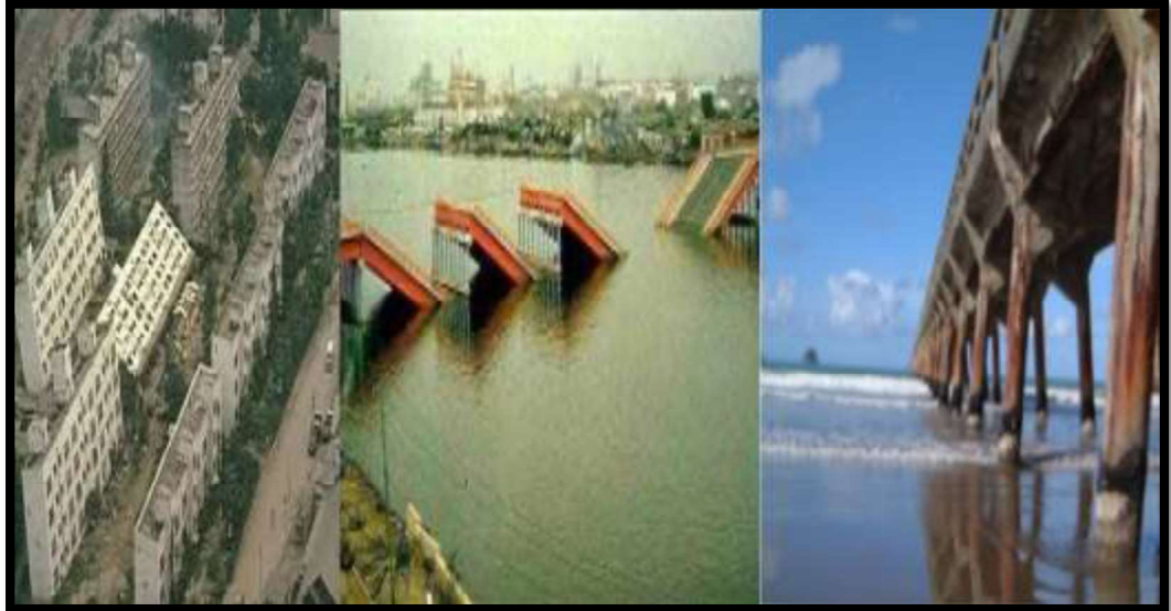
Plate (1.1): Failure of pile foundation due to lateral loads
